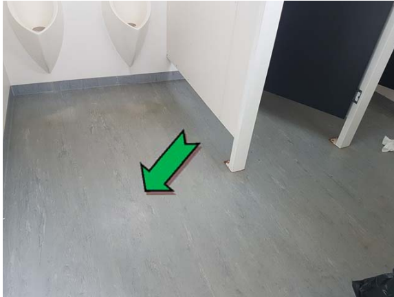
Photo 1. Interior, throughout, floor coverings – non asbestos-containing sheet vinyl.
